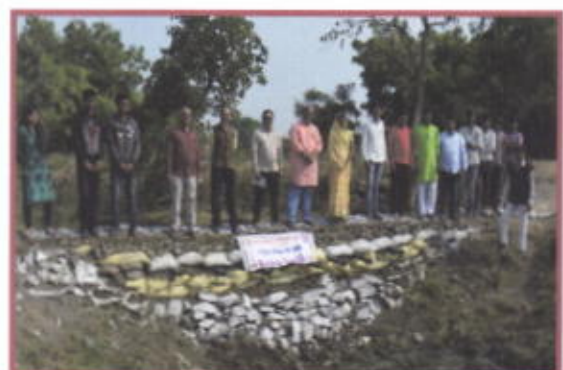
Student created a Bund on water stream
